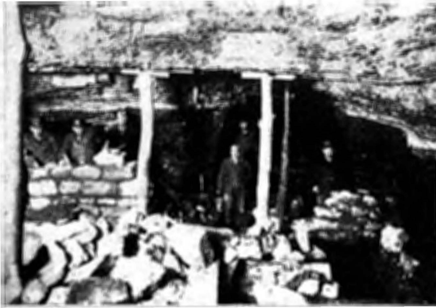
FIG. 3—JOBLESS MINERS, paid with WPA funds, are employed in building these masonry walls used for sealing abandoned coal shafts. The average cost per seal throughout the Appalachian field has been about $40.
